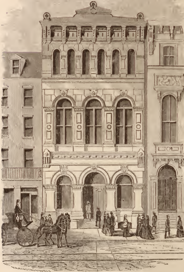
PENNSYLVANIA INSURANCE AND TRUST CO.'S BUILDING.
